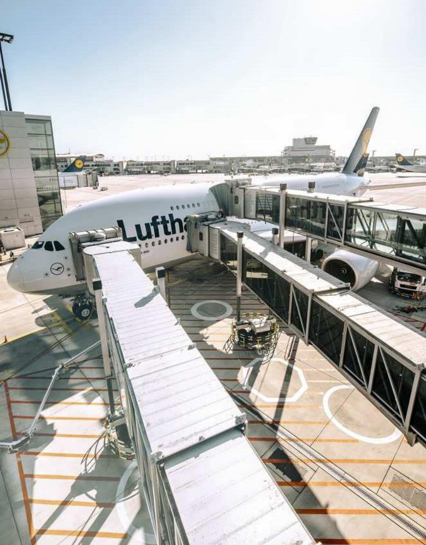
PASSENGER BOARDING BRIDGES
